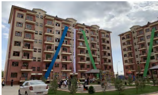
Government affordable houses (Uzbekistan 689 units)
